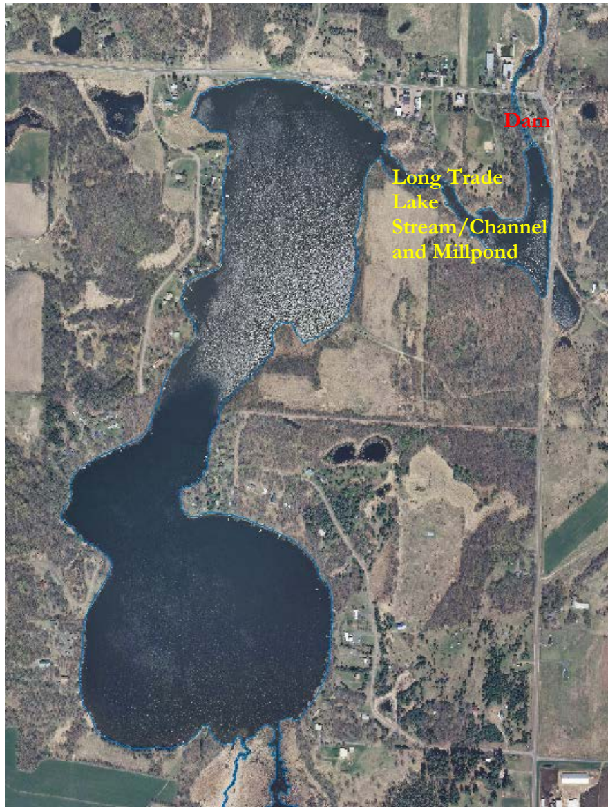
Figure 14: Long Trade Lake Dam, Millpond, and connecting Stream Channel
