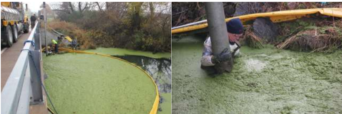
Figure 15: Removal of duckweed and other floating debris from upstream of the Hwy Q Bridge in Lake Como (Photos Courtesy of the BCLA)
