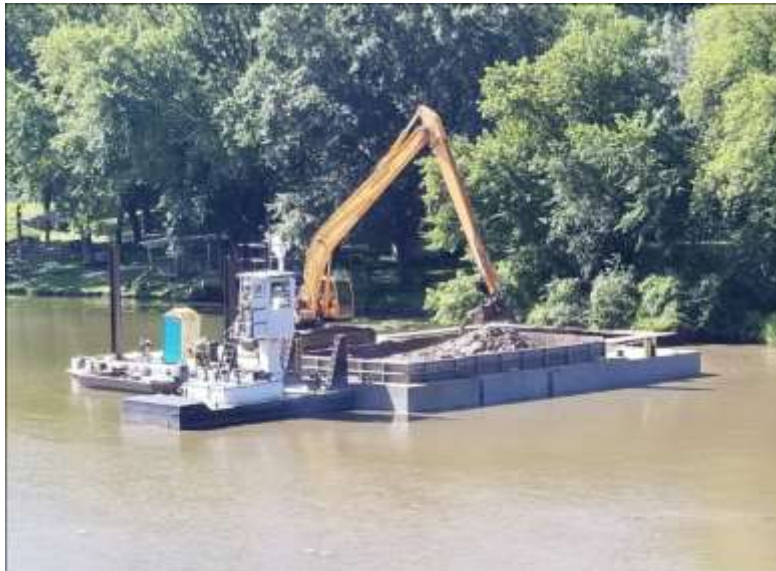
Figure 45: 2019 Dredging operations on Lake Redstone in Sauk County (Photo credit-LRPD)
