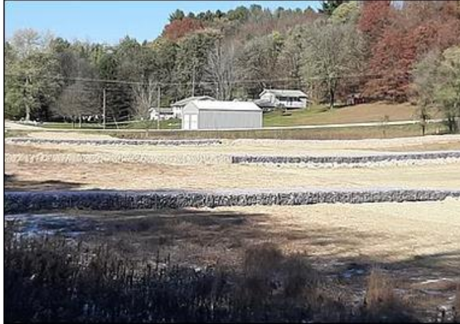
Figure 38: Stone-filled gabion baskets placed at the head of Mourning Dove Bay (LRPD Website)
