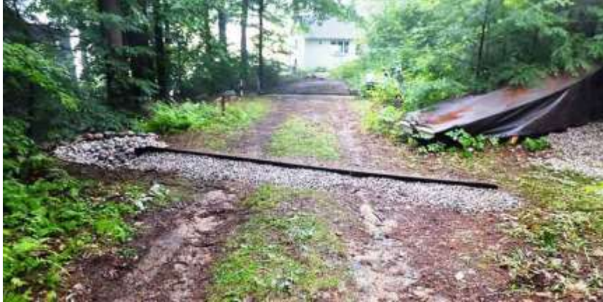
Figure 5: Completed diversion (photo from HealthyLakesWI.com)
