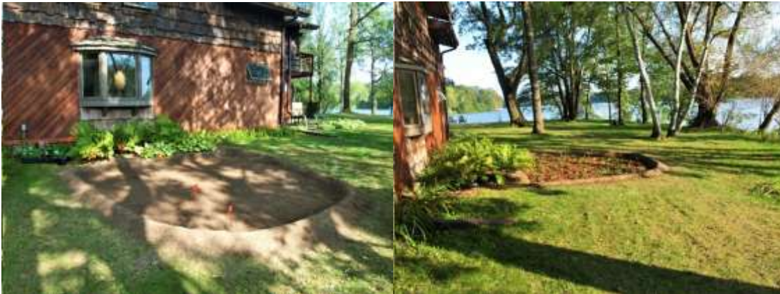
Figure 3: Rain garden installation (left) and upon completion (right).
