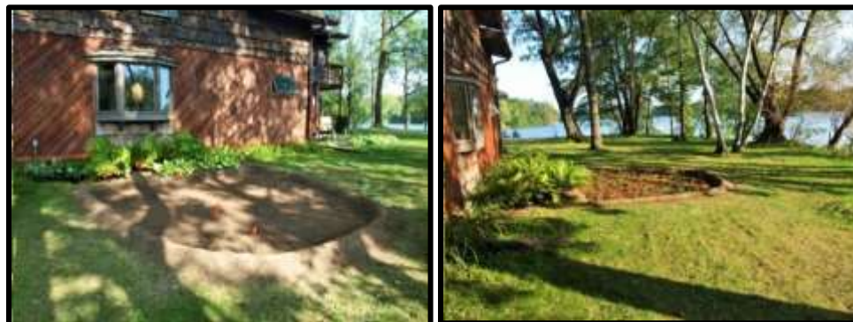
Figure 3: Rain garden installation (left) and completed rain garden (right)
