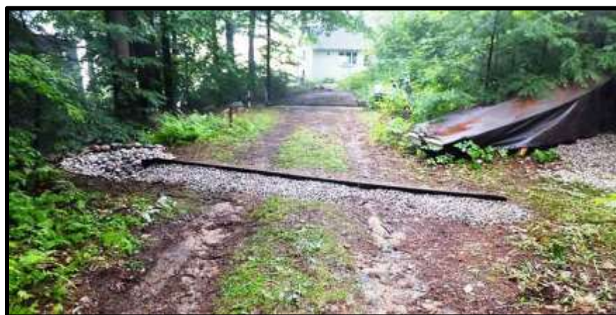
Figure 5: Completed diversion (Photo from HealthyLakesWI.com)
