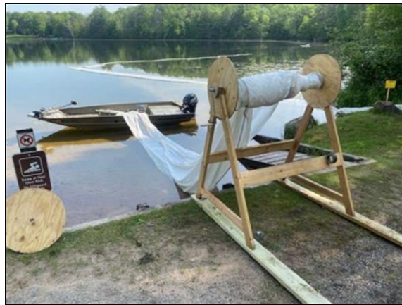
Figure 40. Limno-curtain material on a roll before installation (photo from Marinette Co. LWCD)
