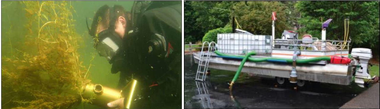
Figure 39. DASH – Feeding EWM into the underwater Suction Hose (Marinette Co.); and a sample DASH Pontoon Boat (Beaver Dam Lake Management District)
