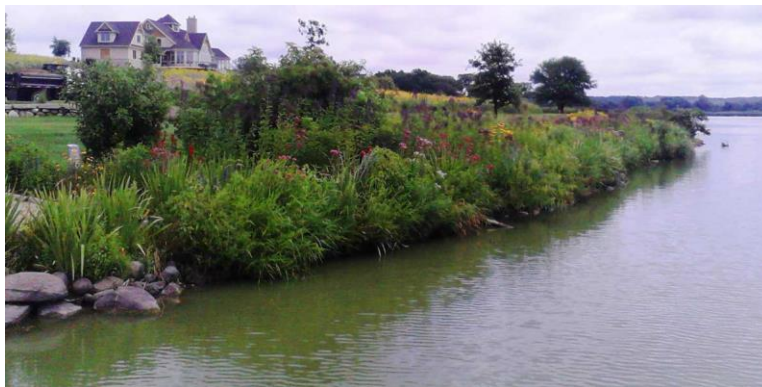
Figure 43: Completed native planting (photo from HealthyLakesWI.com)
