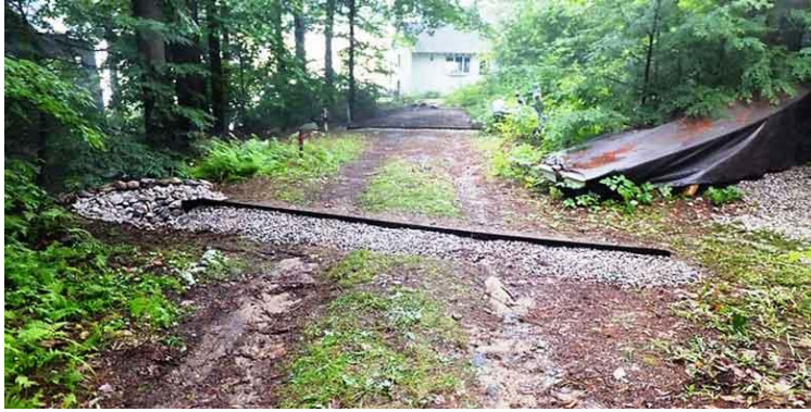
Figure 44: Completed diversion (photo from HealthyLakesWI.com)
